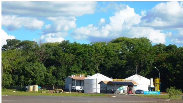
Biomethane pilot plant and filling station © Martin Höher/AEA
