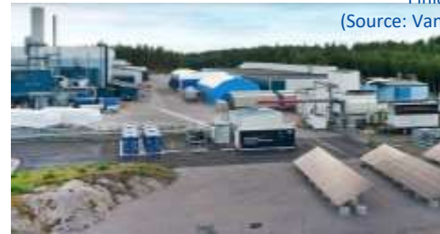
Siemens Energy's Zero Emission Hydrogen Turbine Center (Source: Siemens Energy)
